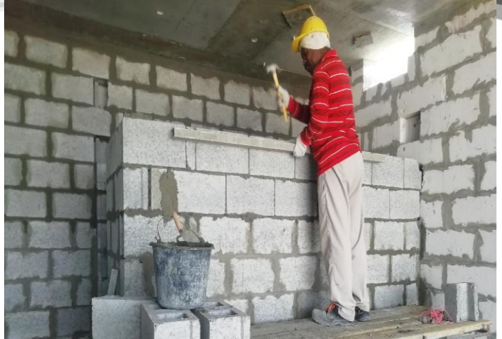
21 st Floor – Block Work
