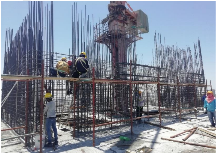
34 th Floor – Steel Work for Shear Wall
