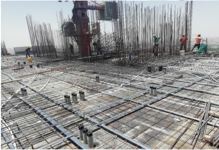
35 th Floor – Steel Work for Slab
