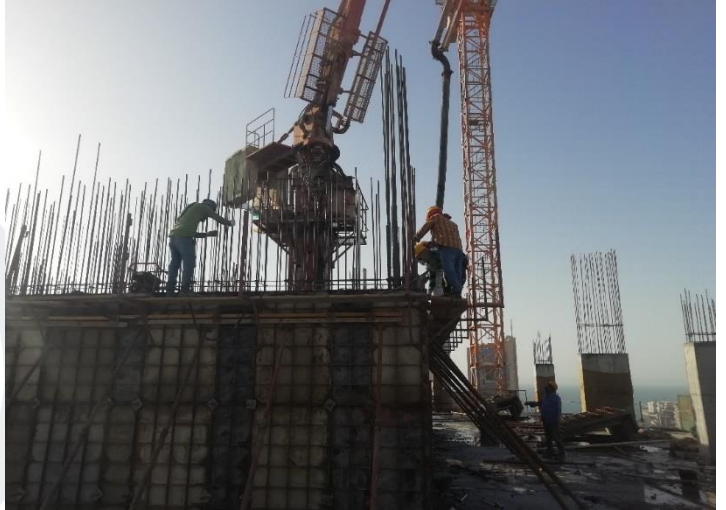
34 th Floor – Concrete Work for Shear Wall
