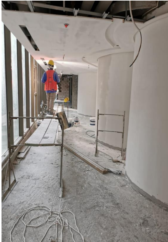
Gypsum Ceiling and Painting Works at Corridor Area (Typical Floor)
