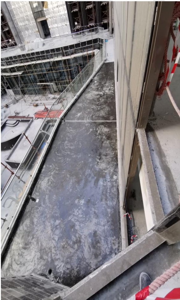
Waterproofing Works & Water Leakage Test for Terrace Area at 1 st Floor
