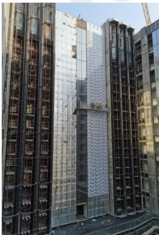
Installation of Aluminum Works (Brackets, Mullion, Rockwool ACP Cladding & Glass and Application of Bitumen Paint)
