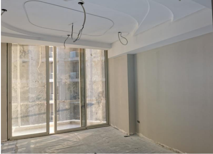
Gypsum Ceiling and Painting Works at Typical Floors
