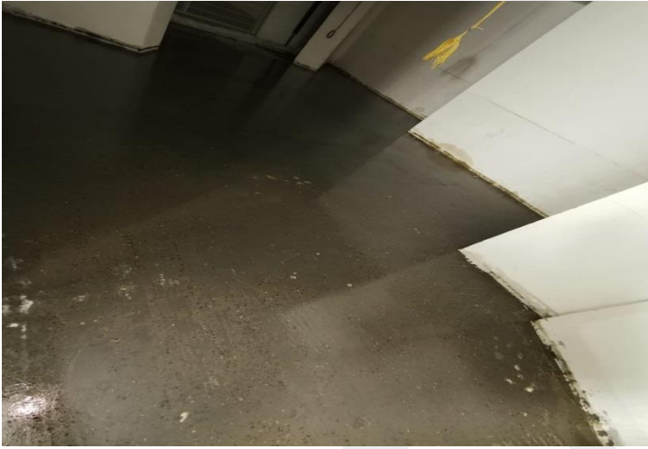
Water Leakage Test at Typical Floors
