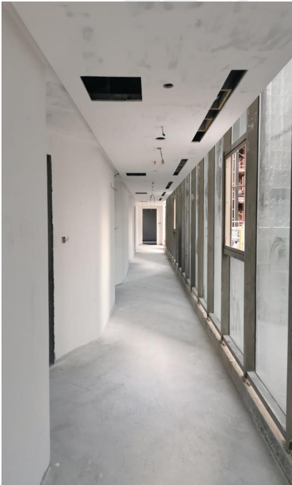
Gypsum Ceiling and Painting Works at Corridor Area (Typical Floor)
