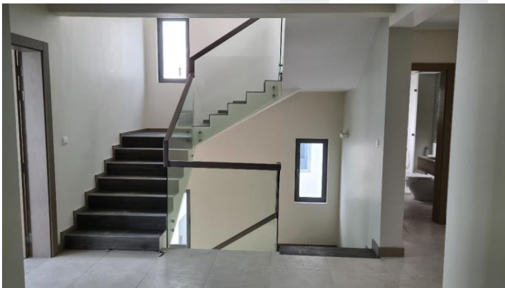
Staircase Handrail Installation in Progress
