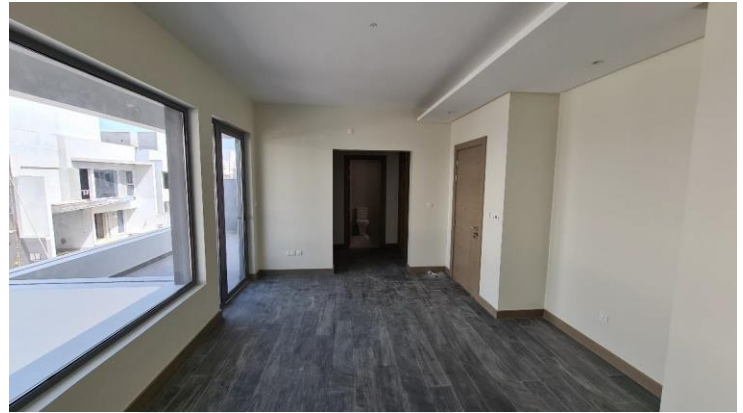
Aluminum Windows Installation in Progress
