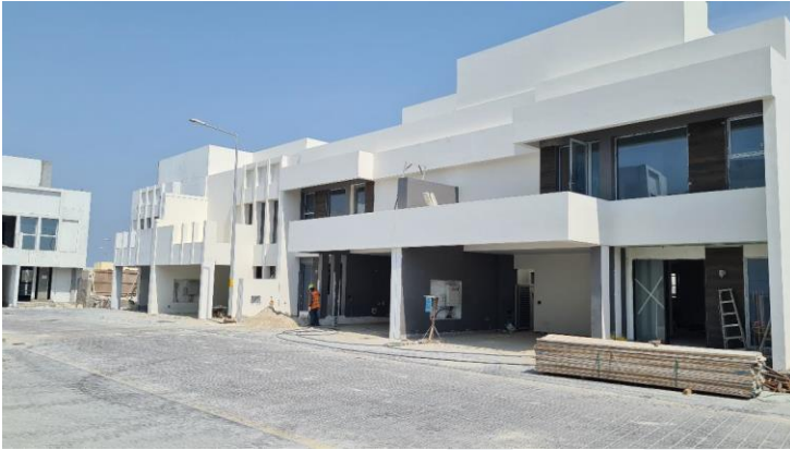
External Painting Works in Progress
