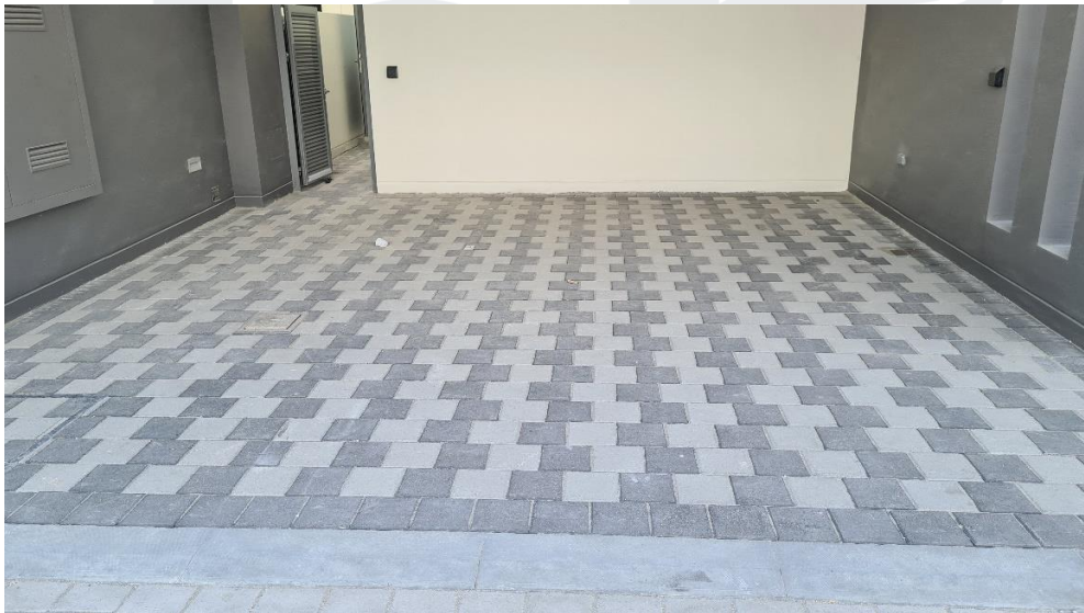
Villas Garage Interlock Installation in Progress
