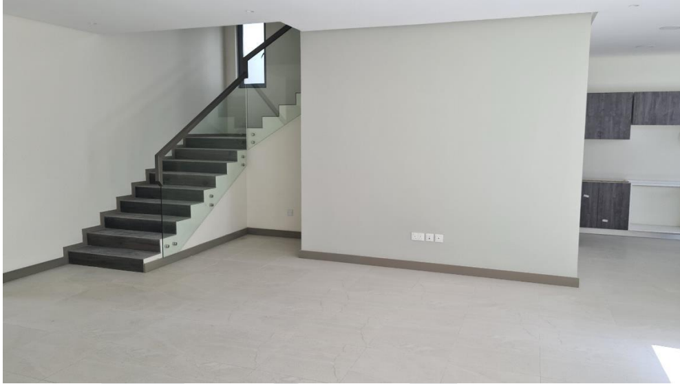
Internal Painting in Progress
