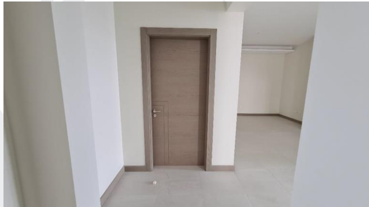
Internal Door Installation in Progress
