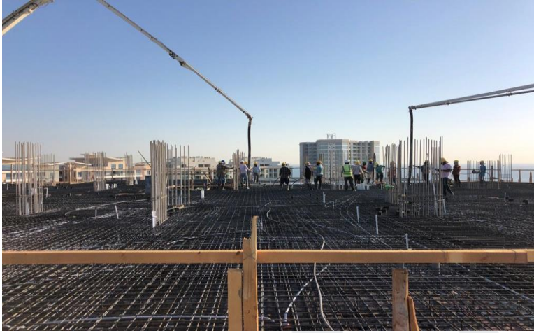
Zone 1 – 6 th Floor Slab and Beam Concrete
