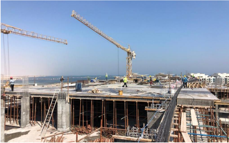
Zone 2 – Roof Slab and Beam Shuttering and Reinforcement Work
