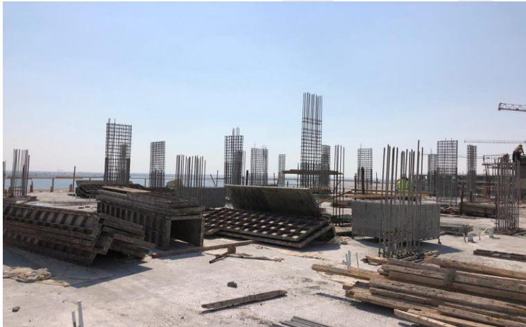
Zone 1 – 6 th Floor Columns Reinforcement Work
