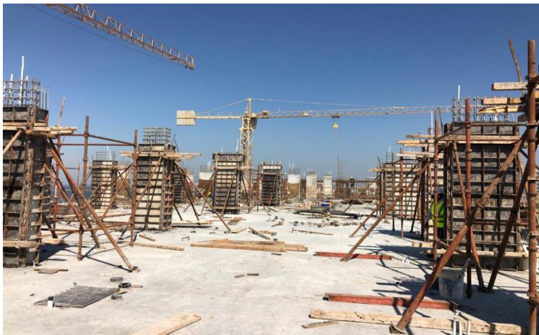
Zone 2 – 6 th Floor Columns Reinforcement and Shuttering Works
