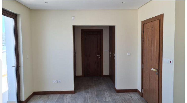
Internal Door Installation in Progress
