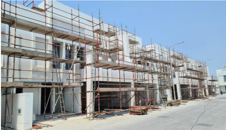
External Painting Works in Progress
