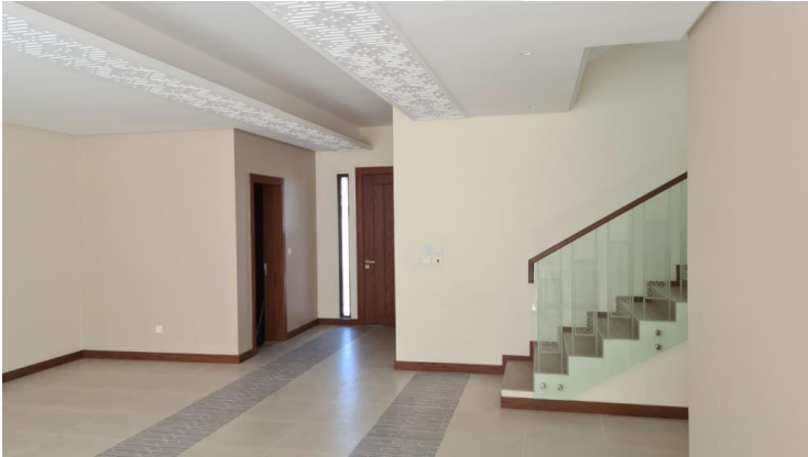
Staircase Handrail Installation in Progress
