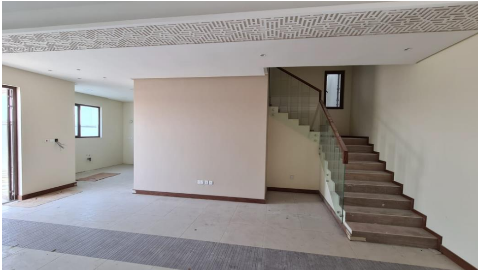
Internal Painting in Progress
