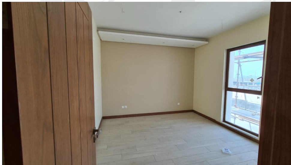
Floor Tile Works Final Finishing in Progress
