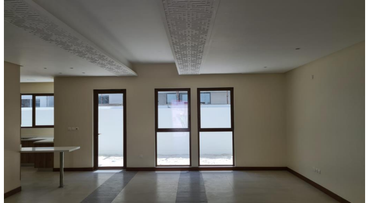
Internal Finishing Works in Progress
