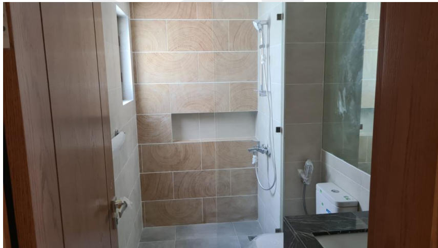
Villa Shower Partition Installation in Progress
