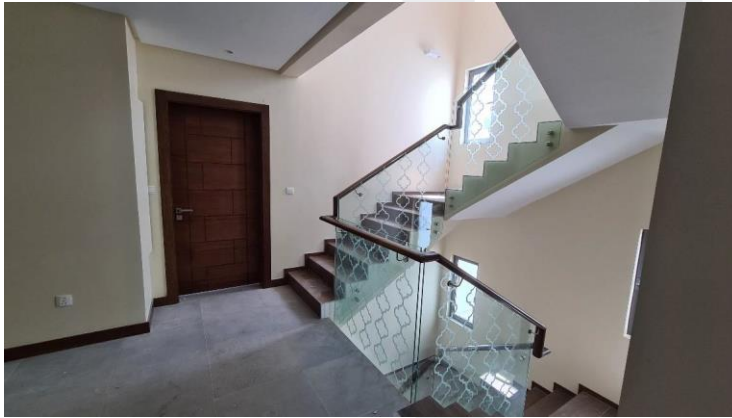
Staircase Handrail Installation in Progress
