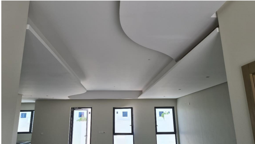
Internal Painting in Progress
