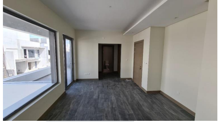
Internal Finishing Works in Progress
