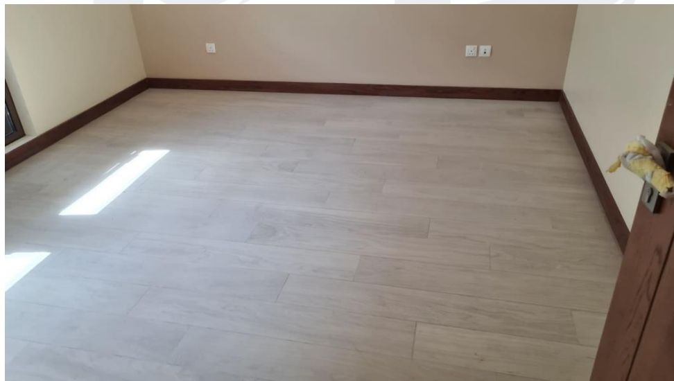
Floor Tile Works Final Finishing in Progress
