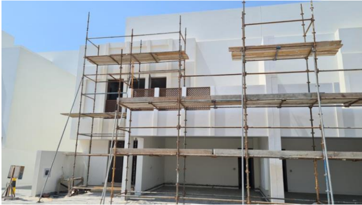
External Painting Works in Progress
