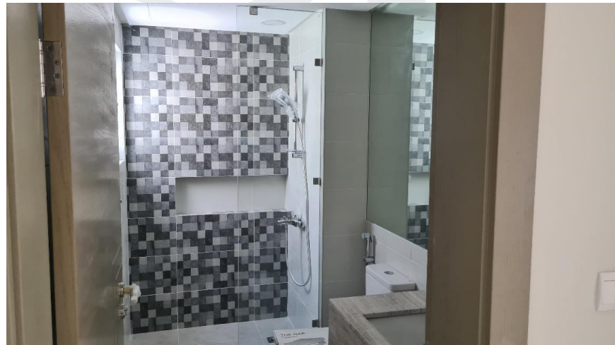
Villa Shower Partition Installation in Progress
