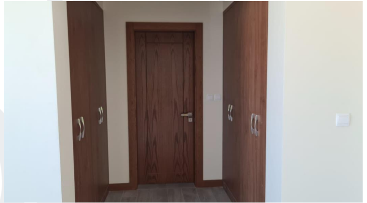
Internal Door Installation in Progress
