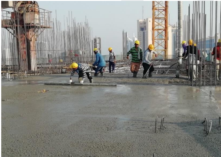
38 th Floor – Concrete Work for Floor Slab
