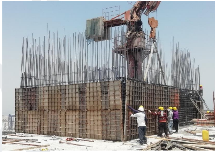
37 th Floor – Shuttering Work for Shear Wall
