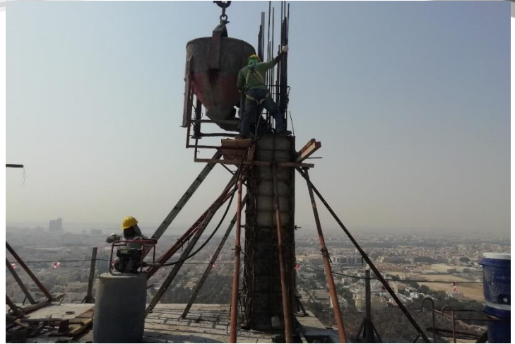
38 th Floor – Concrete Work for Column
