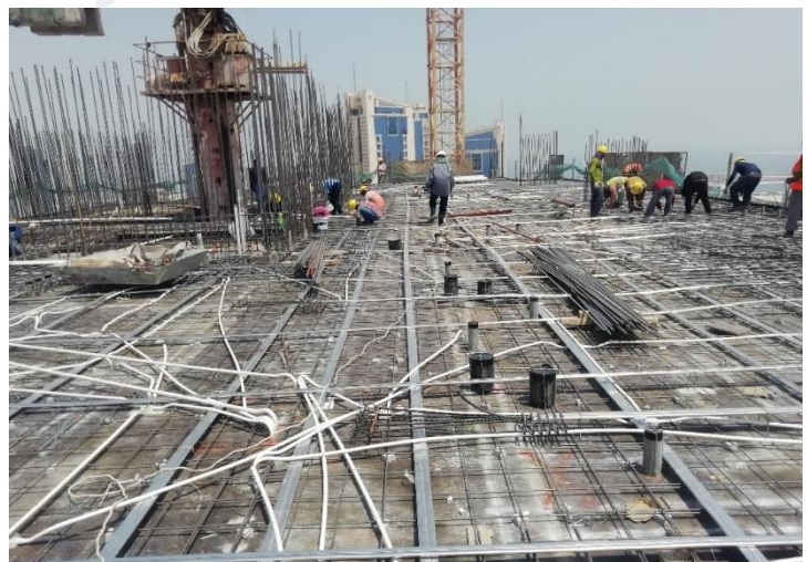
37 th Floor – Steel Work for Floor Slab
