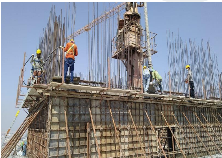
36 th Floor – Concrete Work for Shear Wall
