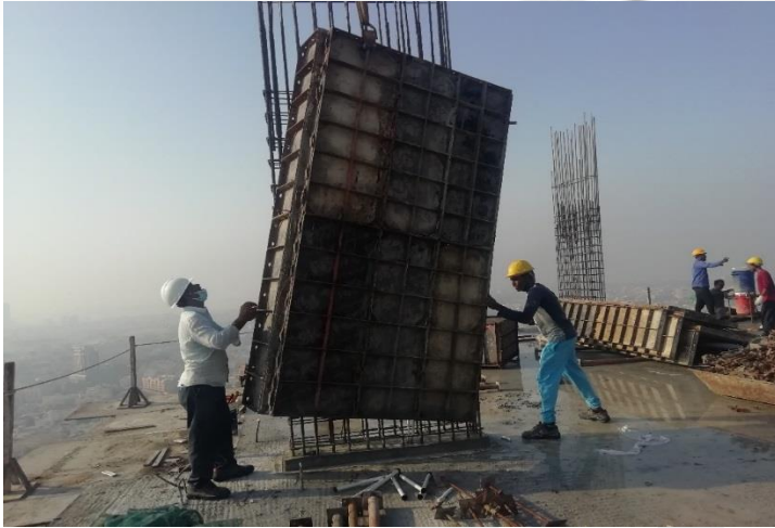
38 th Floor – Shuttering Work for Column
