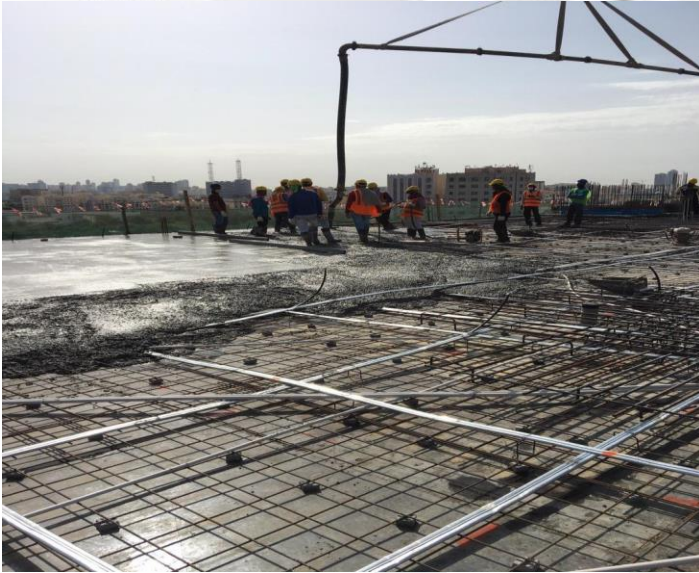
7 th Floor – Slab Concrete Works
