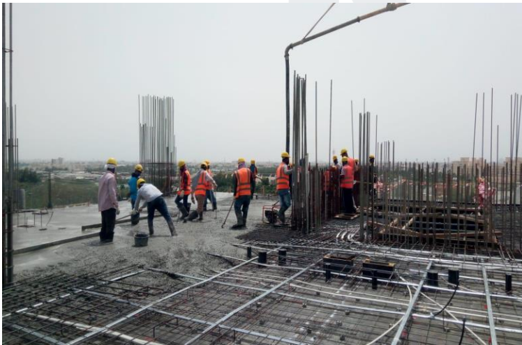
8 th Floor – Slab Concrete Works
