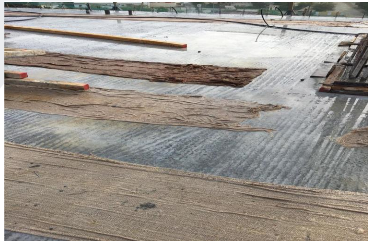
Water Curing Slab
