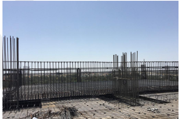
Pool Steel – Reinforcement Works
