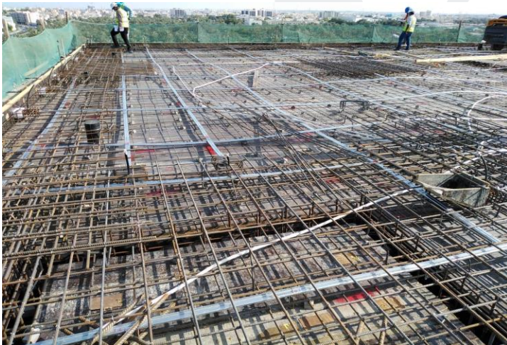
7 th Floor – Swimming Pool Deck Steel Works
