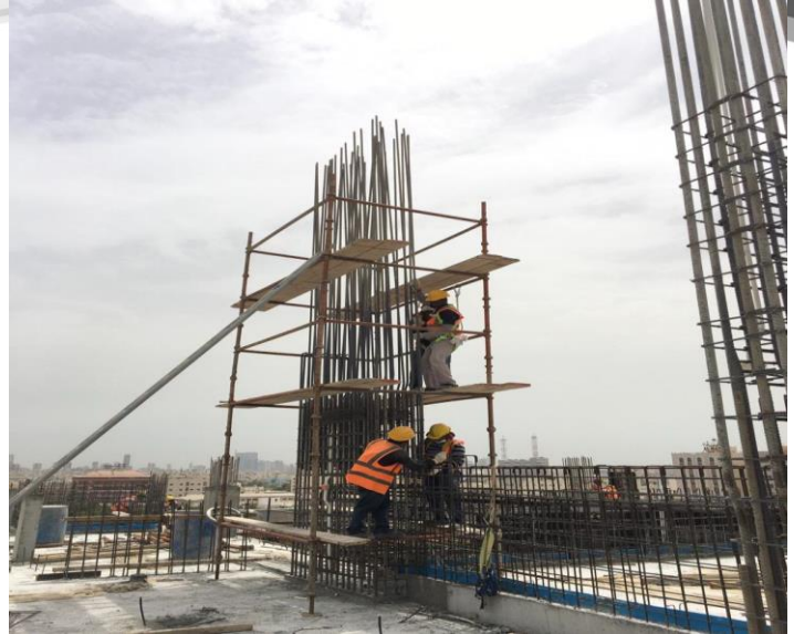
7 th Floor – Column Steel Works
