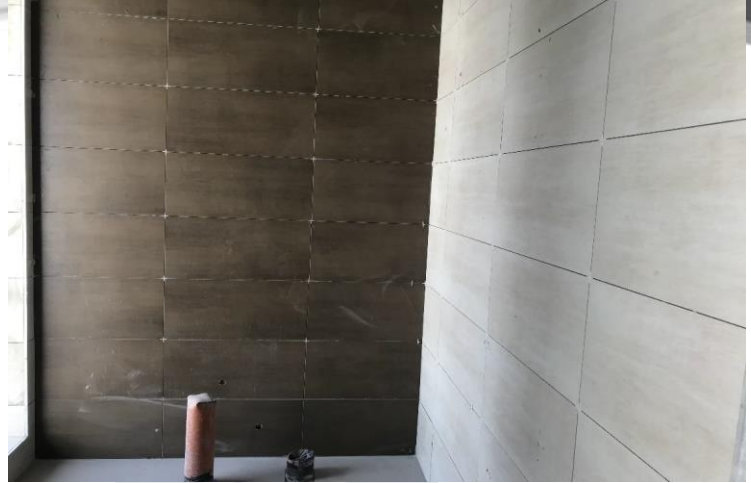
Wall Tiles Fixing in progress.
