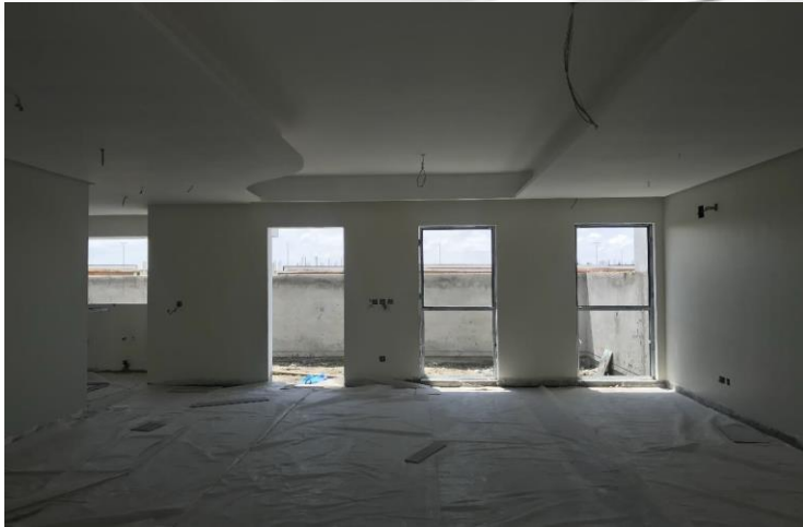
Ceiling Works in progress
