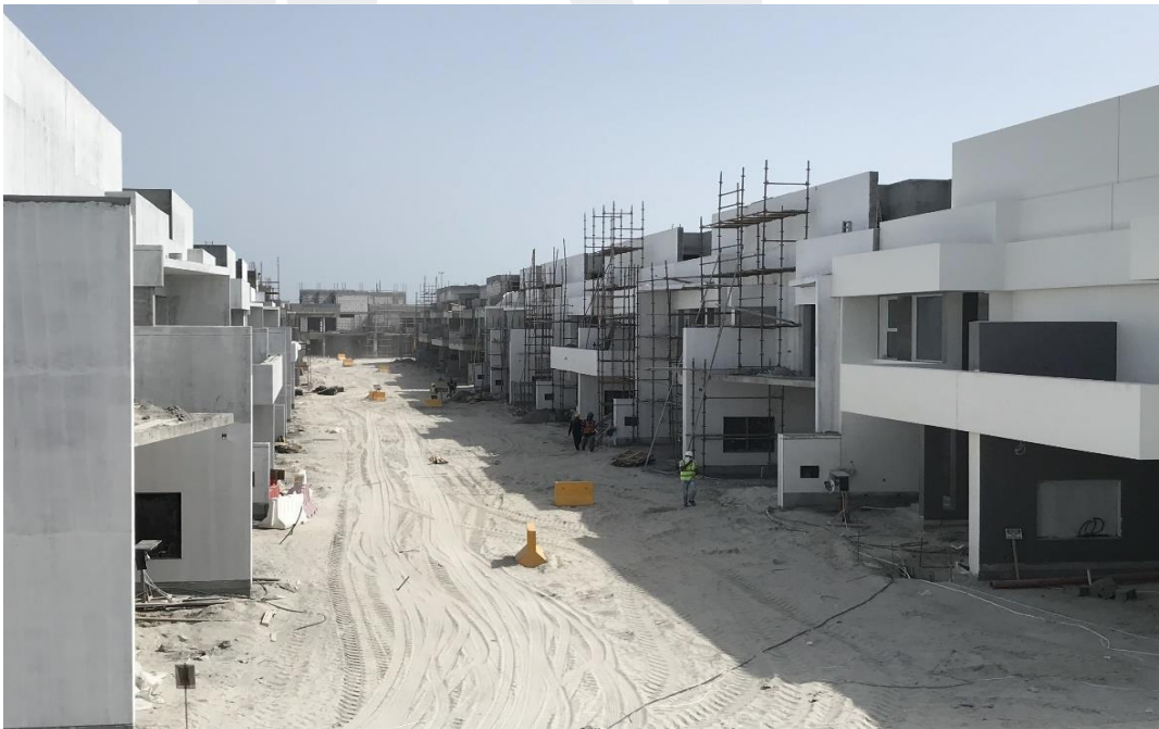
External Painting works in progress
