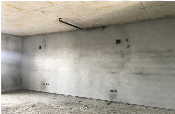
Internal Plastering Works in progress
