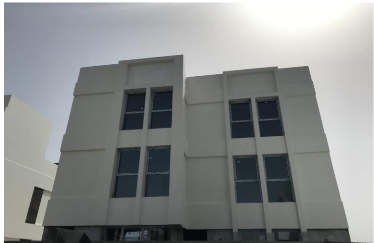
Aluminum Installation Works in progress
