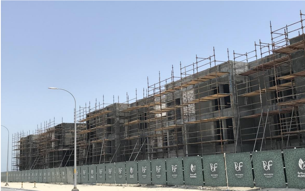
Plastering Preparation works in progress
