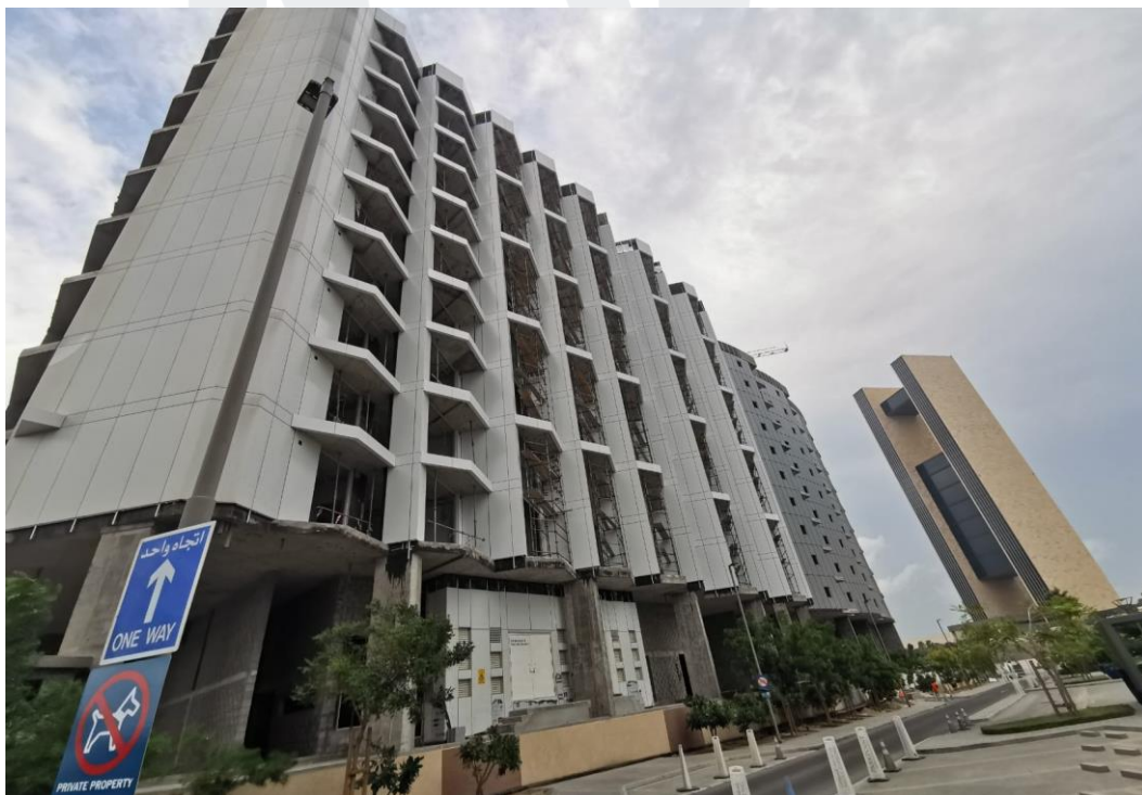
Installation of Aluminum Works (Brackets, Mullion, Rockwool ACP Cladding & Glass and Application of Bitumen Paint)
