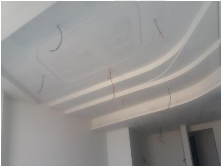
Gypsum Ceiling and Painting Works at Typical Floors
