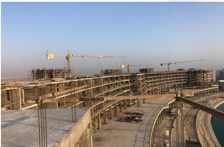
Upper Roof Columns and Slab Shuttering Work
