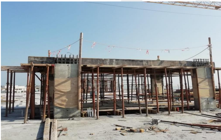
Zone 1 & 2 – Upper Roof Slab and Beam Concrete Work
