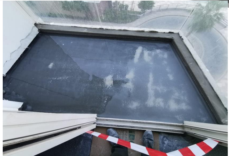
Waterproofing Works for Balcony Area
