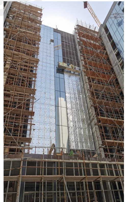
Installation of Aluminum Works (Brackets, Mullion, Rockwool ACP Cladding & Glass and Application of Bitumen Paint)
