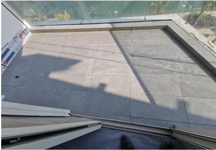
Marble Works for Balcony Area at Typical Floors
