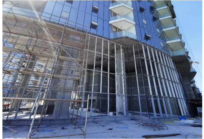
Installation of Aluminum Works (Brackets, Mullion, Rockwool ACP Cladding & Glass and Application of Bitumen Paint)
