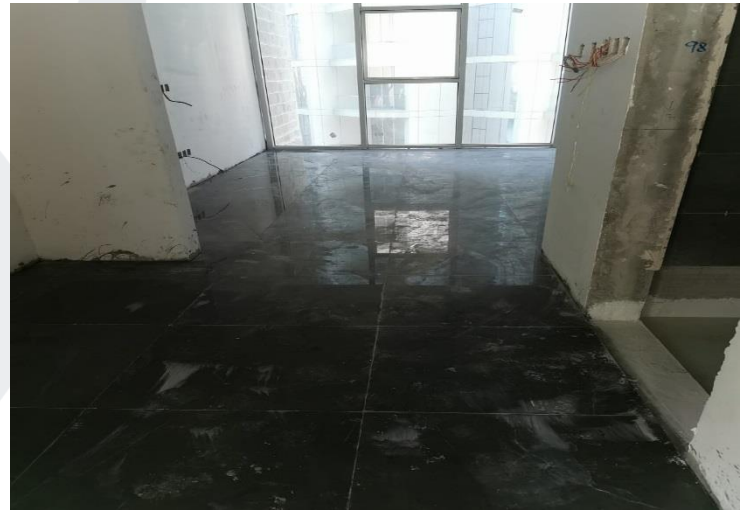
Marble Floor for Flats at Typical Floor
