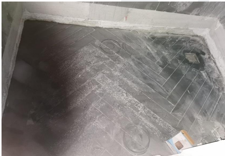
Marble Floor Works for Toilet at Typical Floors
