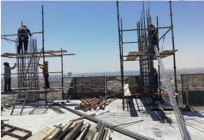
33 rd Floor – Steel Work for Column
