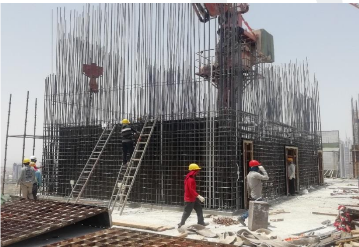
32 nd Floor – Steel Work for Shear Wall
