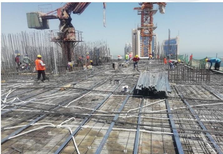
32 nd Floor – Steel Work for Slab
