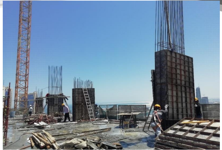
33 rd Floor – Form Work for Shear Wall
