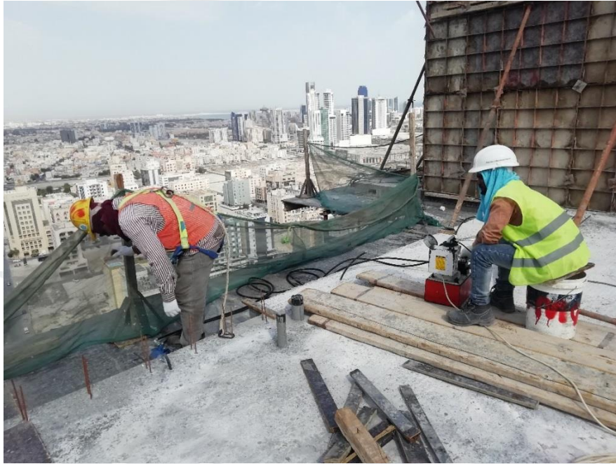
32 nd Floor – Slab PT Stressing Work
