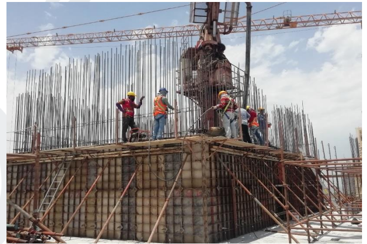
32 nd Floor – Concrete Work for Shear Wall
