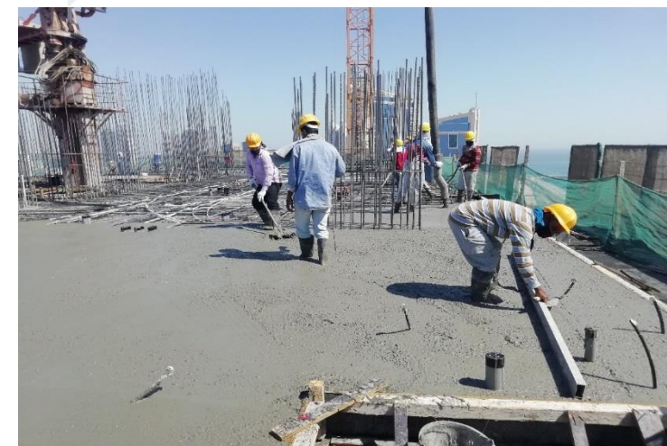
33 rd Floor – Concrete Work for Slab
