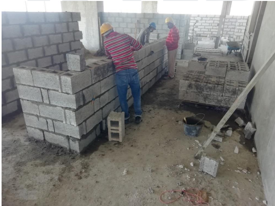
20 th Floor Block Work
