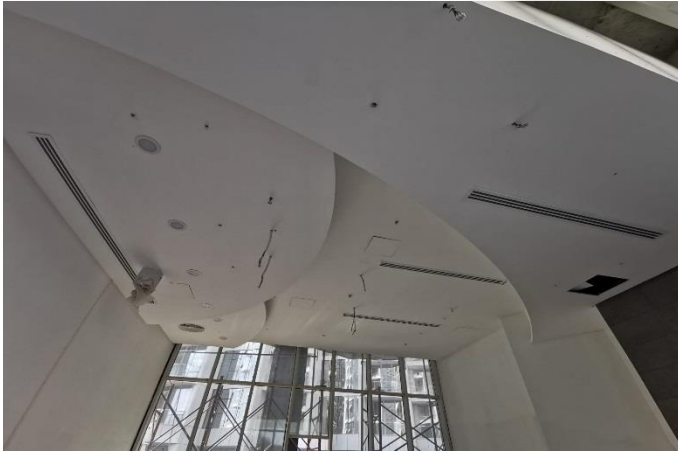
Gypsum Ceiling Works at Ground Floor
