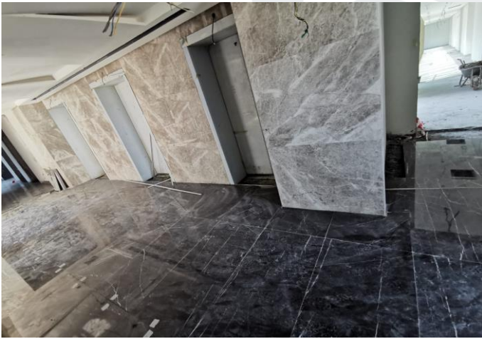
Marble Cladding Works at Typical Floors
