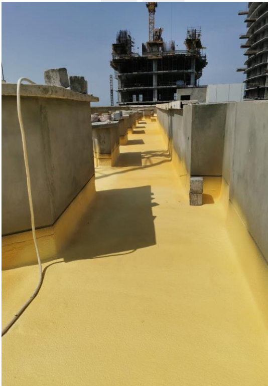
Application of PU Foam at Roof Floor
