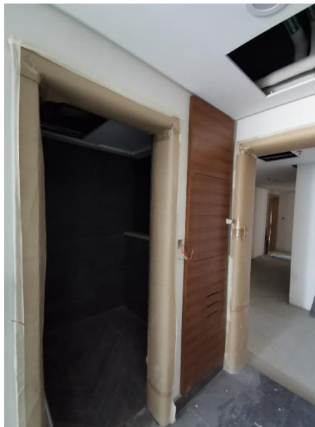
Fixing of Doors at Typical Floors
