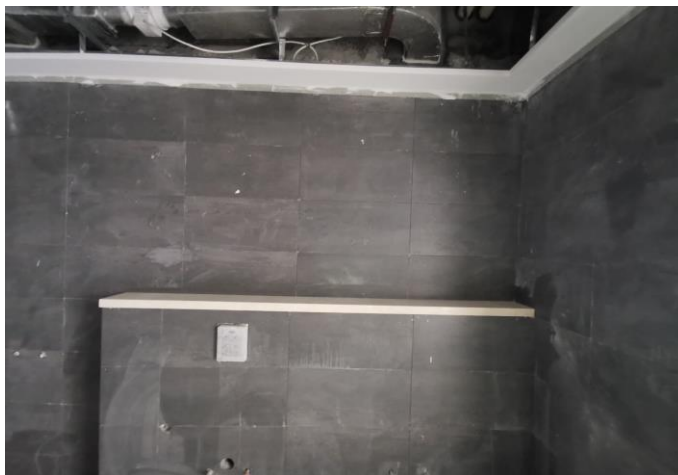
Tile Works for Bathroom at Typical Floors
