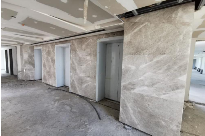
Marble Wall Cladding Works for Lift Lobby Area at Typical Floors
