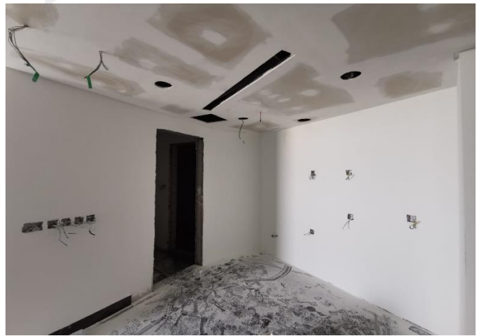
Application of Paint for Walls & Ceiling at Typical Floors
