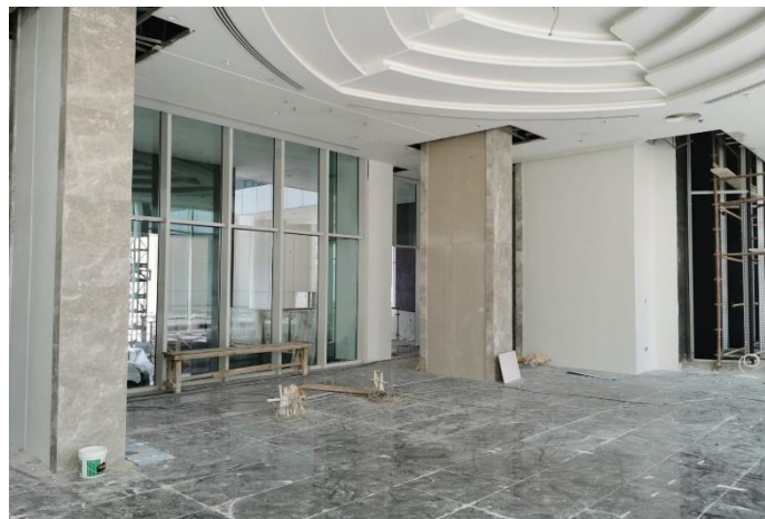
Fixing of Marble Wall Cladding works at Ground floor Reception Area
