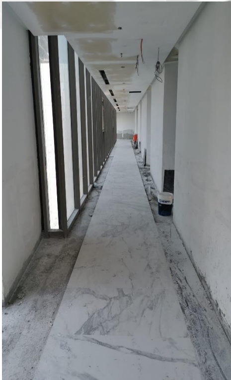
Fixing of Marble & Tiles in Corridor Area and Fixing of Marble Wall Cladding at GF Reception Area
