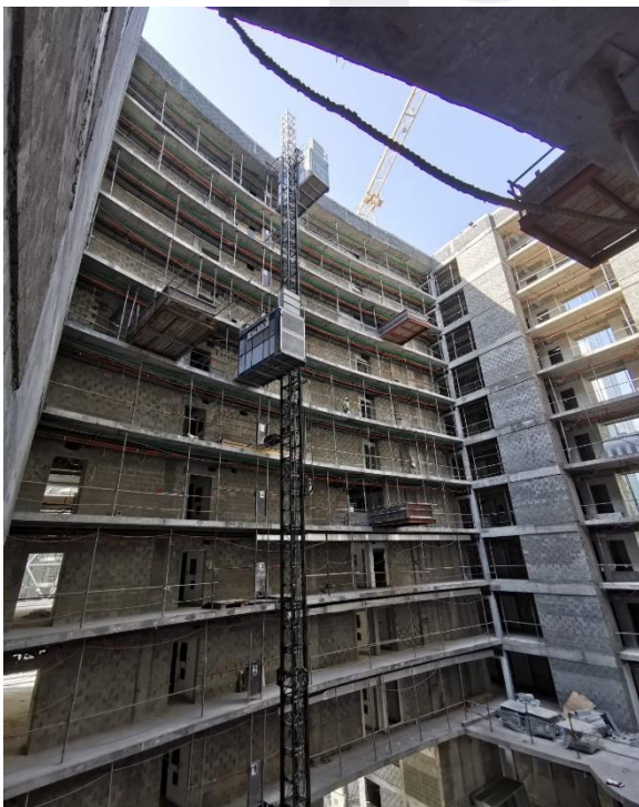
Installation of Aluminum Work (Brackets, Mullion, Rockwool, ACP Cladding and Glass and Application of Bitumin Paint)
