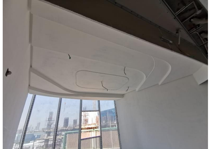
Gypsum Ceiling Works at Typical floor
