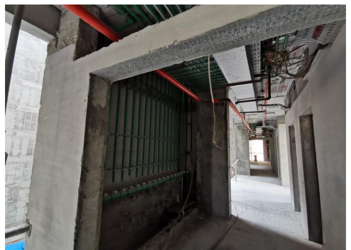
Installation of MEP Services at Typical Floor
